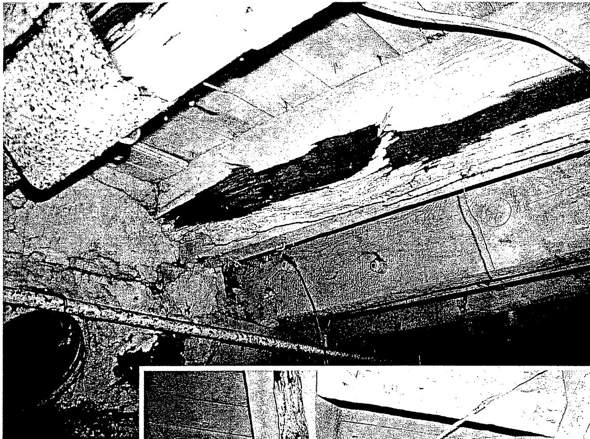
Damaged Framing
